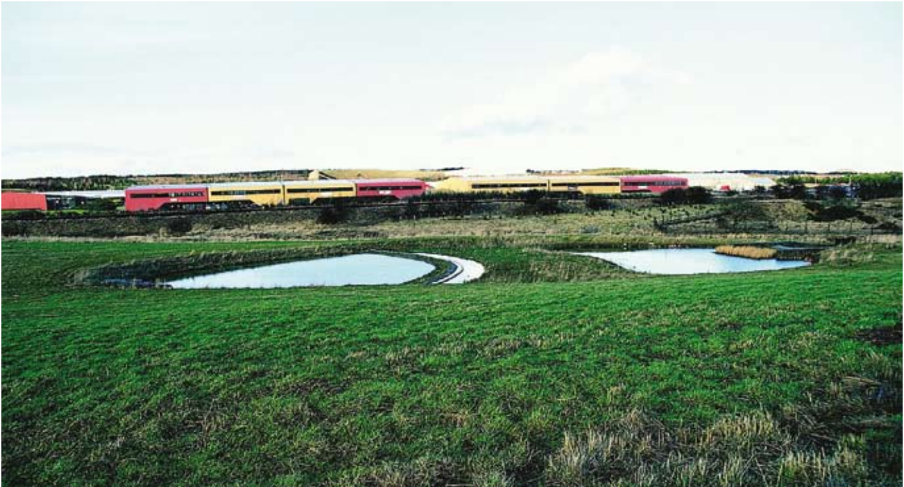
This picture shows a filter strip that has been integrated into the pond design in Livingstone. The gravel filter strip produces a rooting medium for plants between the two sections of the pond.
