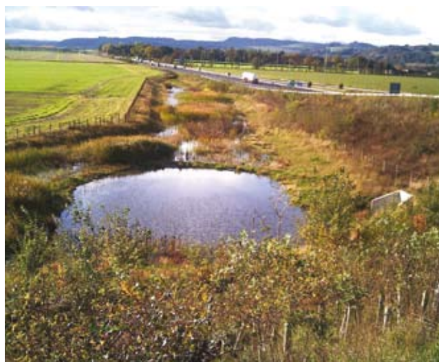
Retention pond beside the A92, Dundee.
