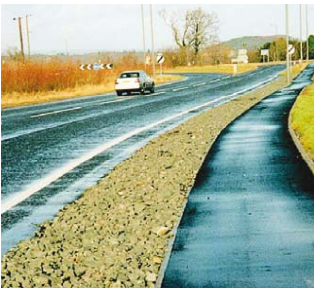
A filter drain at the edge of a road in Stirling. There are no kerbs or gullies incorporated into the design.
