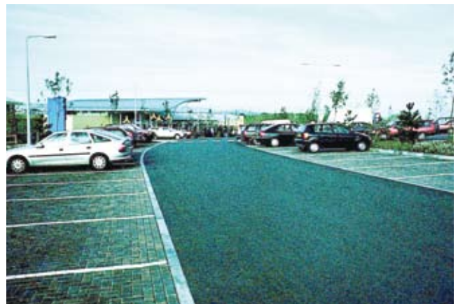
The parking bays at this motorway service area has been built with porous blocks. The rainfall from the tarmac access roads runs onto these bays.
