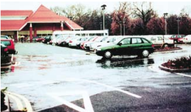
Porous paving of the parking area, at a supermarket in Wokingham, Berkshire, is clearly visible.
