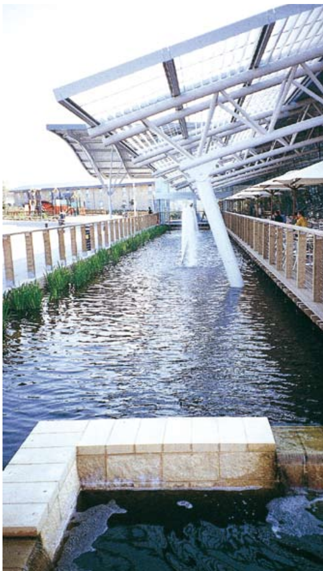
Water features can be incorporated into both rural and urban settings to improve amenity value. Roof water from the site flows to this attractive water feature at the Wheatley Services Area on the M40.
