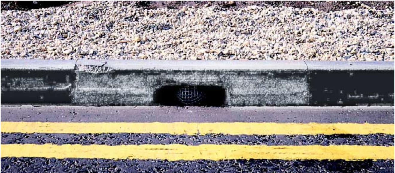
Infiltration trench at the edge of a minor road. Water is taken into the trench via off-let kerbs.
