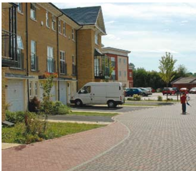
Water is collected and drained beneath the permeable paving in this residential area (Photograph provided by Oxfordshire County Council).
