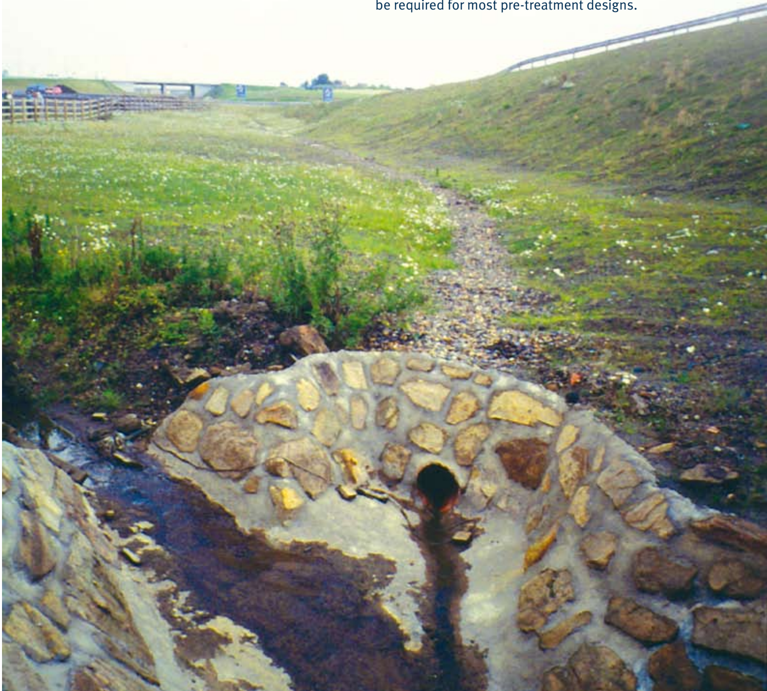
This infiltration trench is incorporated into the landscape areas on a road embankment. The trench has an overflow into a stream.
