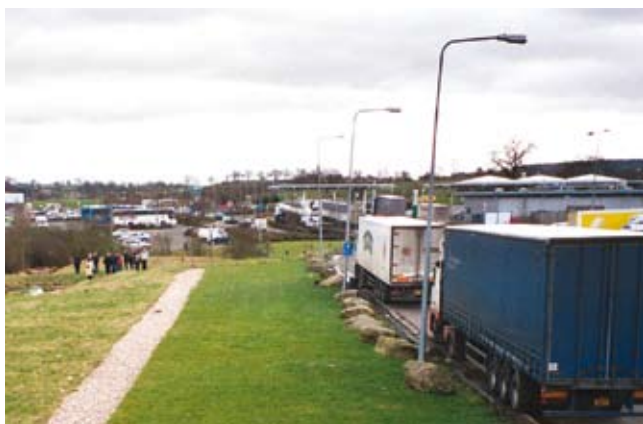
Drainage from a lorry park crosses a filter strip to an infiltration trench at this site in the Midlands.
