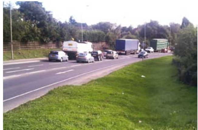
Swale on A8000 near Edinburgh. No kerbs or gullies are required.
